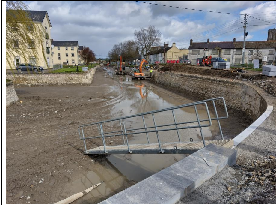
Extensive restoration of canal harbour walls
